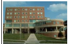
Hutchinson Hall and the Carlson Library
