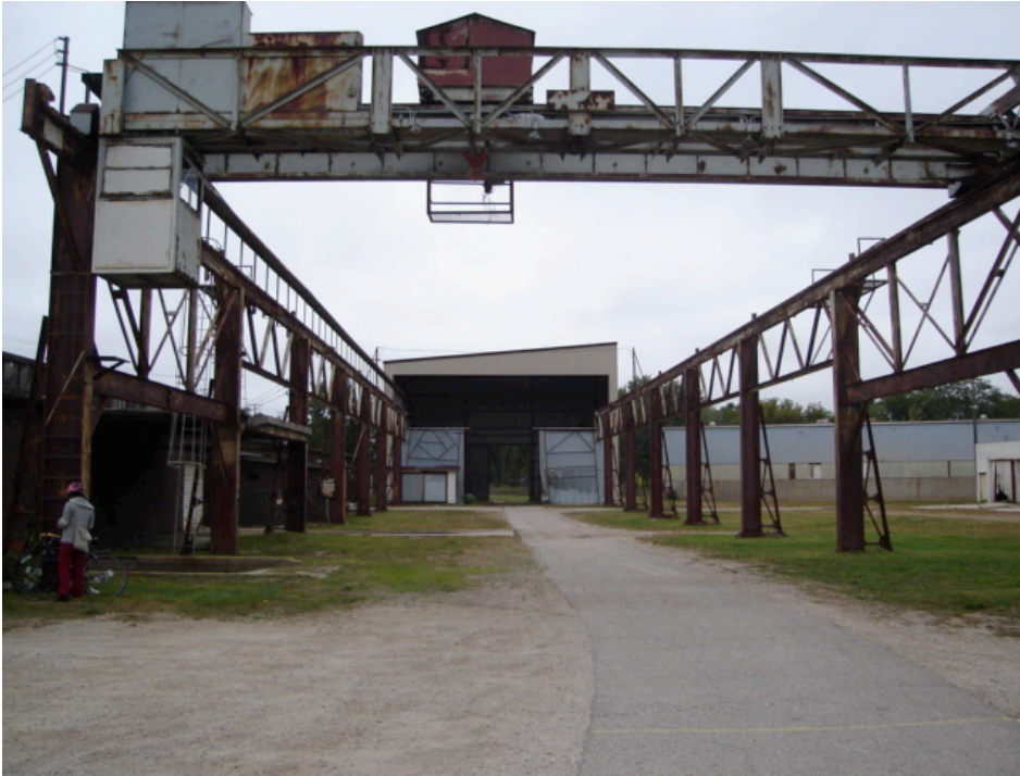
Figure 6: Exterior view, Kupfer Center. Madison, WI
