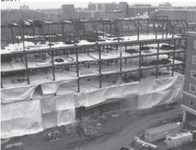
New Biomedical Engineering building under construction on the University of Rochester campus
