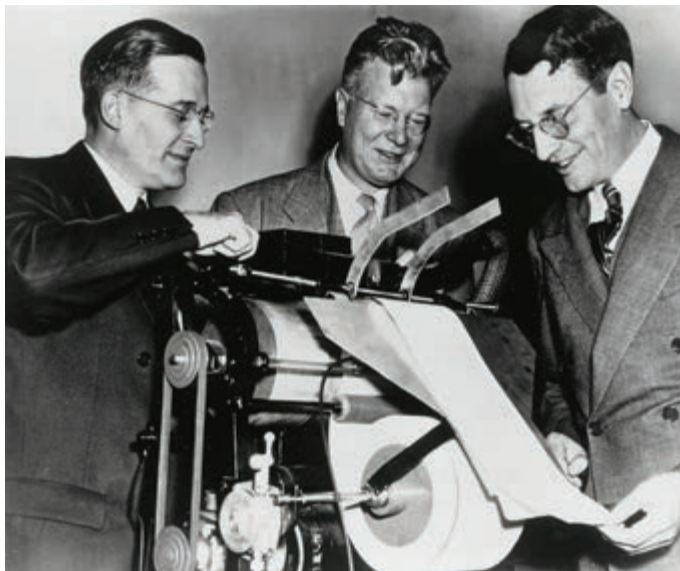
ROLLOUT: Haloid's John Dessauer, Carlson, and Wilson test an experimental xerography machine at the Battelle Institute in 1948.
